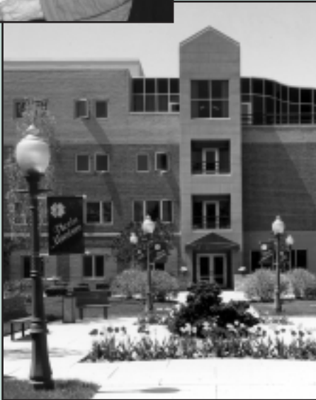
The David A. Miller Assisted Living Community adjacent to Phoebe Home allows residents who need help with some, but not all aspects of daily living to remain independent in modern apartments. The Miller Family Fund was created to provide charitable care to those whose personal resources have run out.
